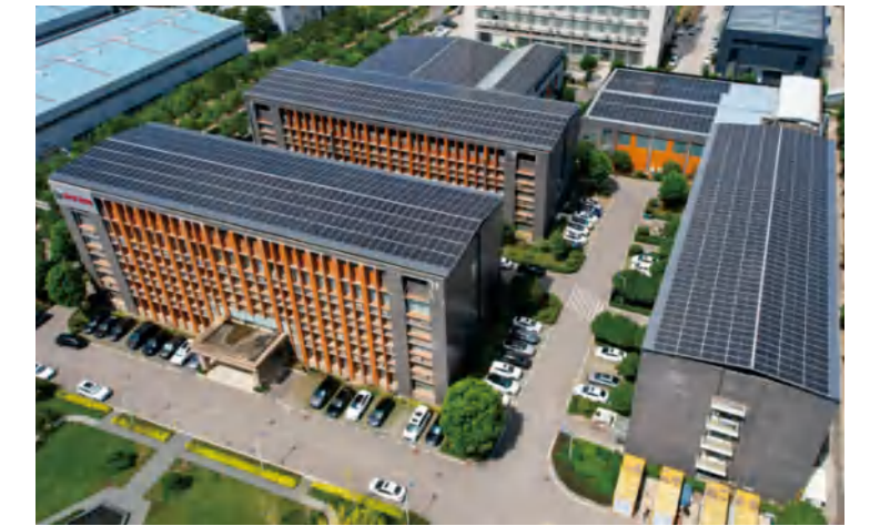
Rooftop photovoltaic (PV) installation at the Wuhan campus
