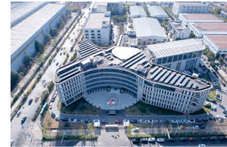
Rooftop photovoltaic (PV) installation at the Wuhan campus
